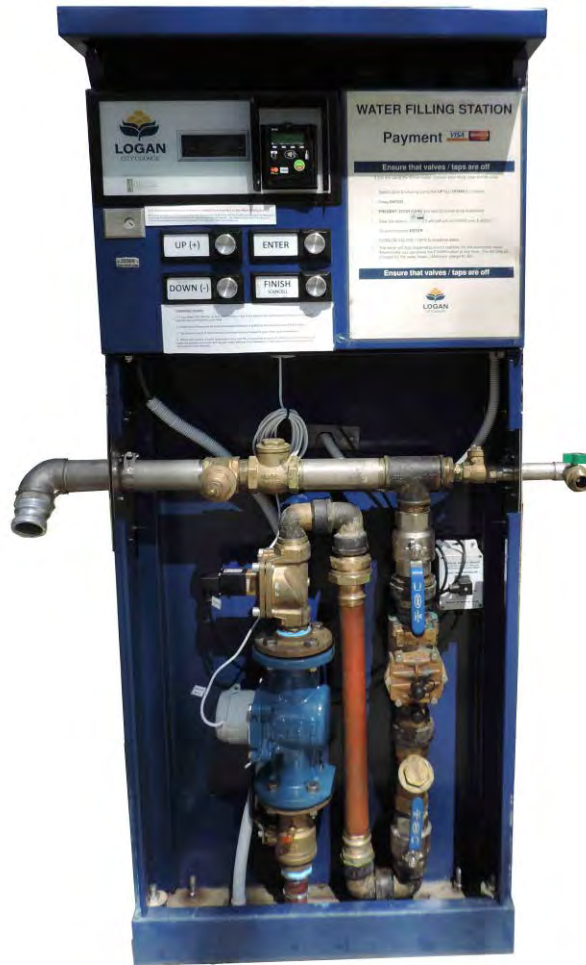
Figure 4 - WD2500 with internal backflow prevention
