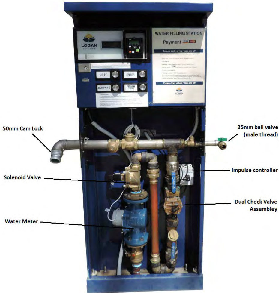
Figure 8 - WD2500 with internal backflow prevention
