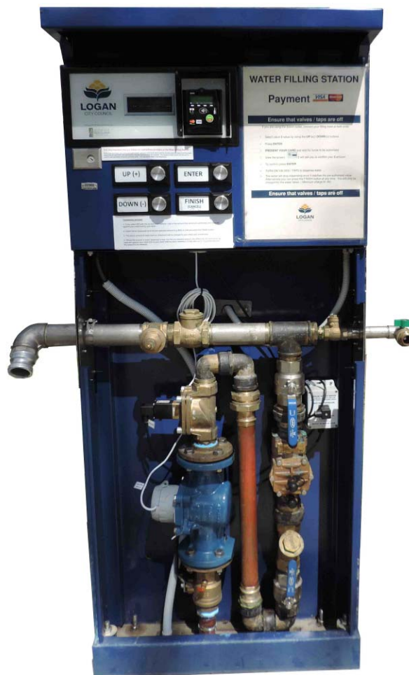
Figure 4 - WD2500 with internal backflow prevention
